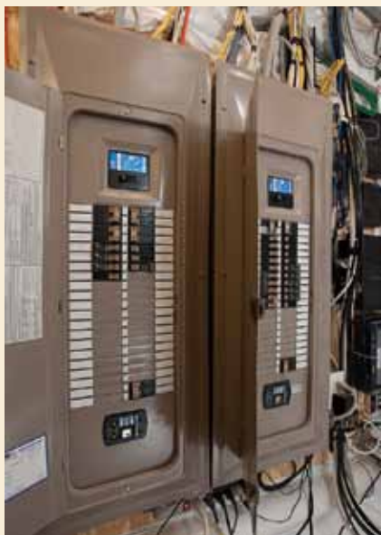
CH Load Center with surge protection provided by EATON CORPORATION.
